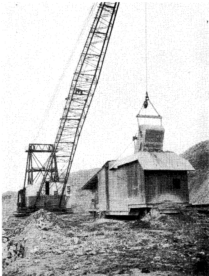
Fig. 2. Eight cu.yd. bucket discharging blasted rock into mobile crushing plant.
