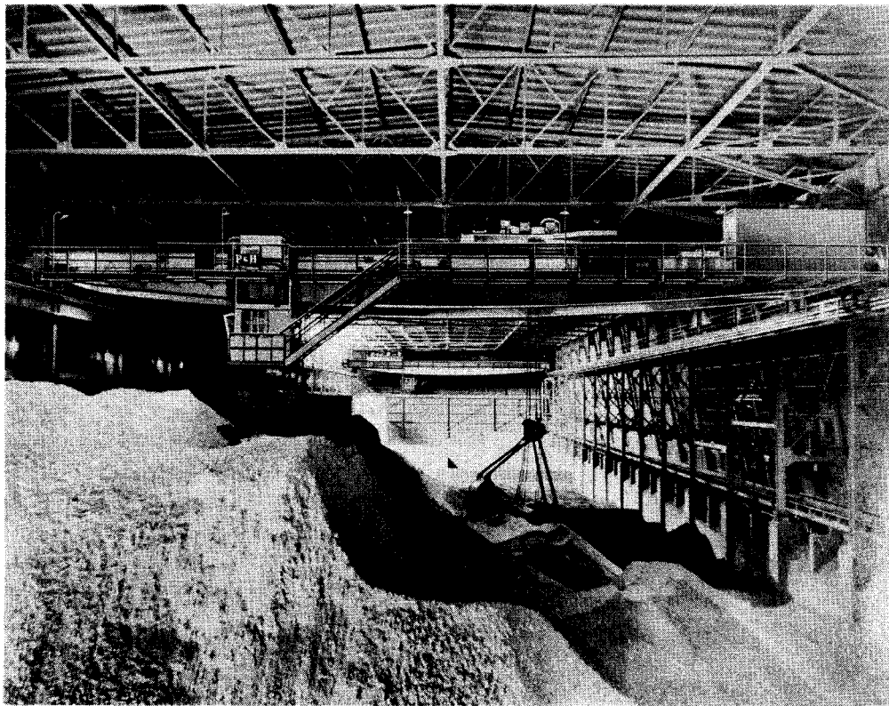
Figure 4. Enclosed Storage Building of the Prospect Hill Plant.
