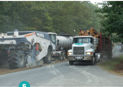
5 Mixing cement and water into pulverized pavement as traffic runs in the adjacent lane.
