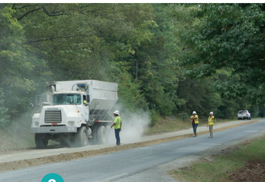
Calibrated spreader places Portland Cement at the appropriate rate.
