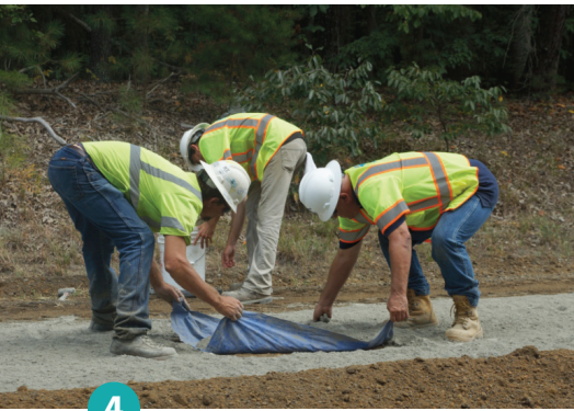
4 Testing technicians check cement spreader rate using a square yard tarp.
